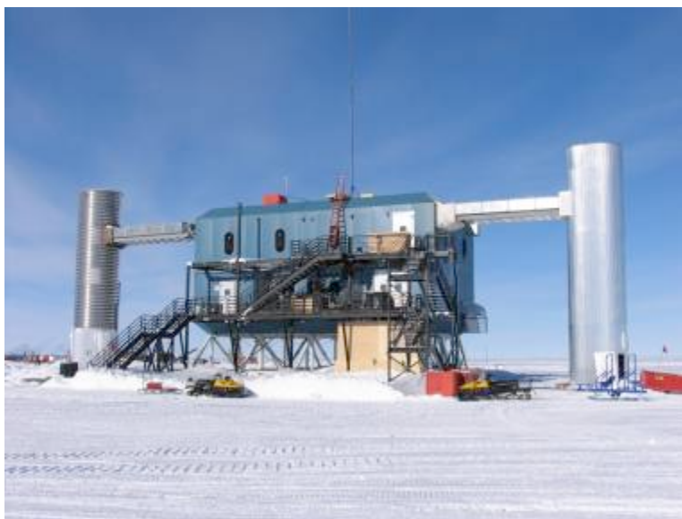
Figure 3.2-1. IceCube Laboratory (ICL). The ICL at the South Pole houses the online computing system which is critical to mining data from IceCube.
